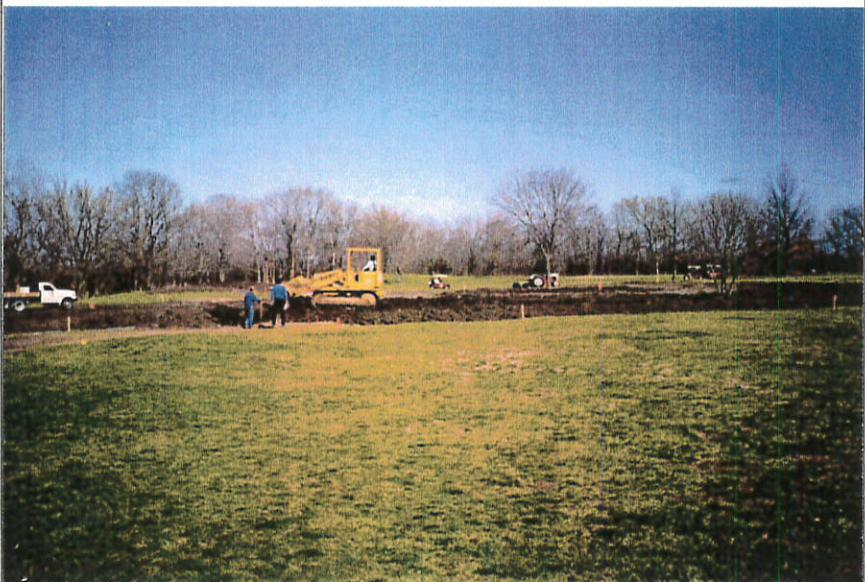
Cap construction over exposed battery landfill debris
