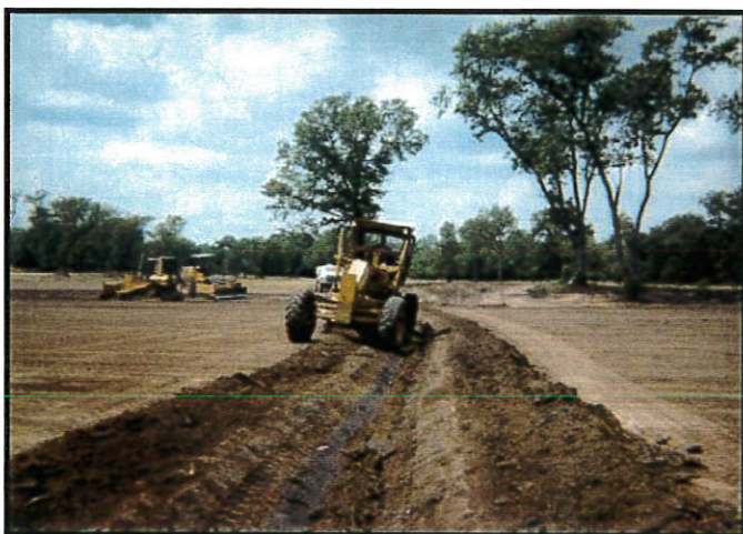
Construction of drainage swale.
