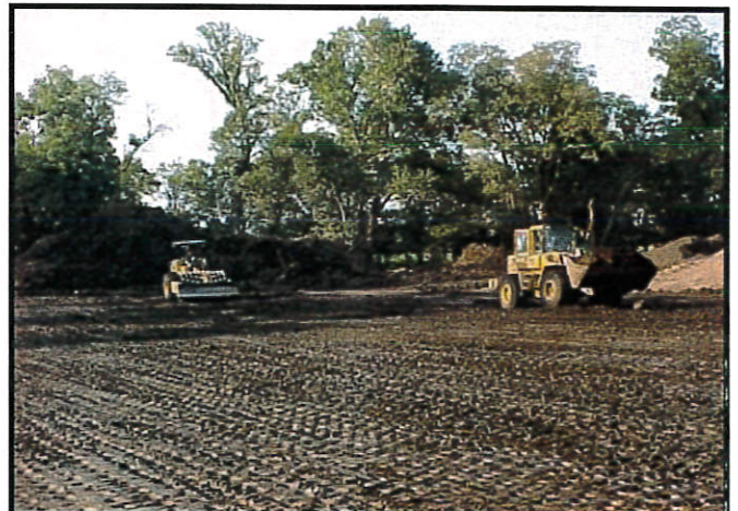
Placement and compaction of clay cap.
