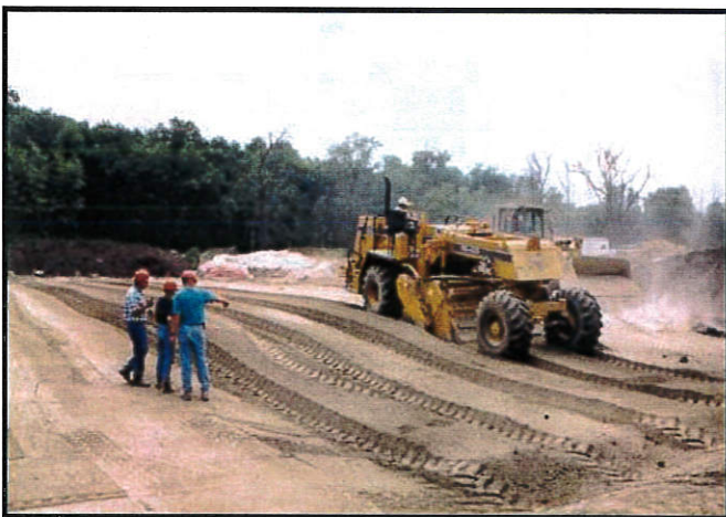
Stabilization of sludge waste. Impacted soils mixed with cement kiln dust to raise pH and demobilize subsurface waste.
