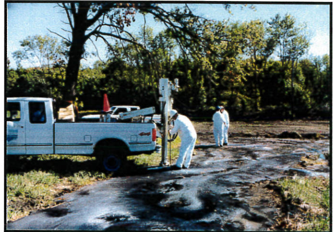
Sampling and characterization of sludge material.
