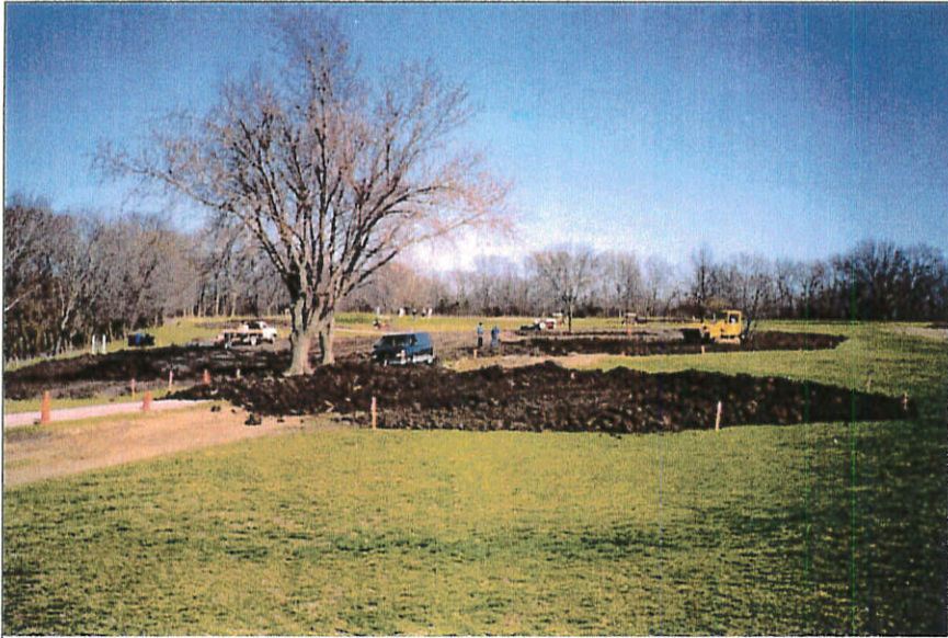
Cap construction over exposed battery landfill debris
