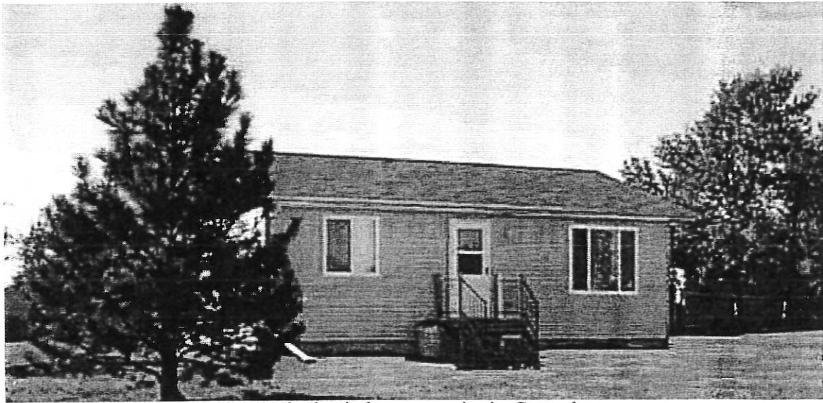
Here's the basic house on site in Gettysburg
