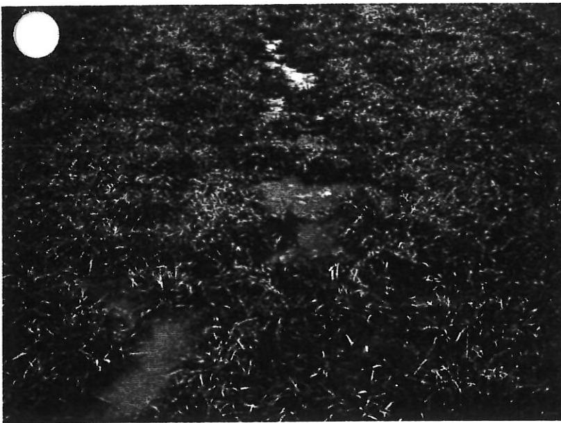
Poor filter strip maintenance. Equipment was used on the filter strip when wet, which led to channelization.
