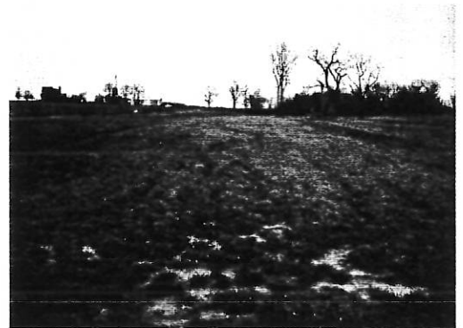
Uniform, level slope across a filter strip.
