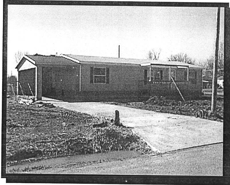
Photo 2-New Manufactured Home under Construction 25 th and Briggs-Parsons, Kansas
