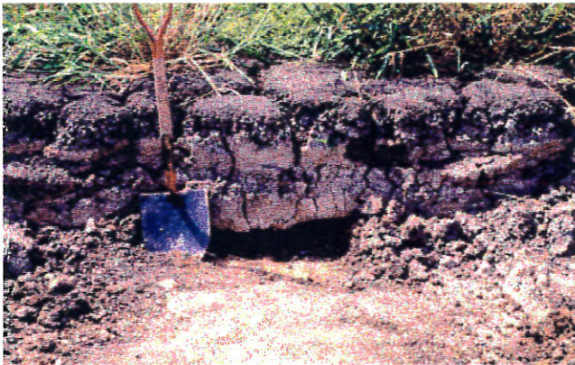
Above: Organic sludge layer that has been deposited along the sides and bottom of a cattle feedlot runoff lagoon. Photo taken when lagoon was emptied for cleaning.
