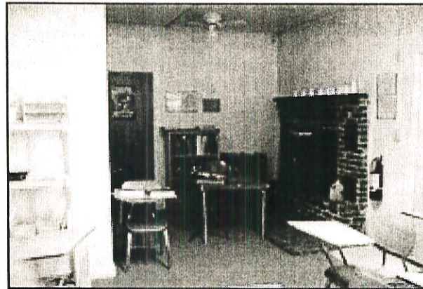
Main classroom and entrance to teacher's office
