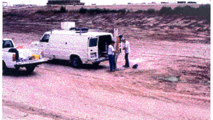
Right: Collecting soil cores from an 11-year-old lagoon using a direct-push soil probe. The lagoon had been dried and sludge removed prior to sampling.
