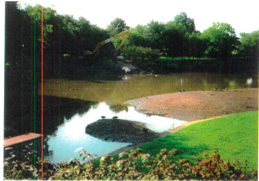
Small basin with siltation and dredging from the shore.
