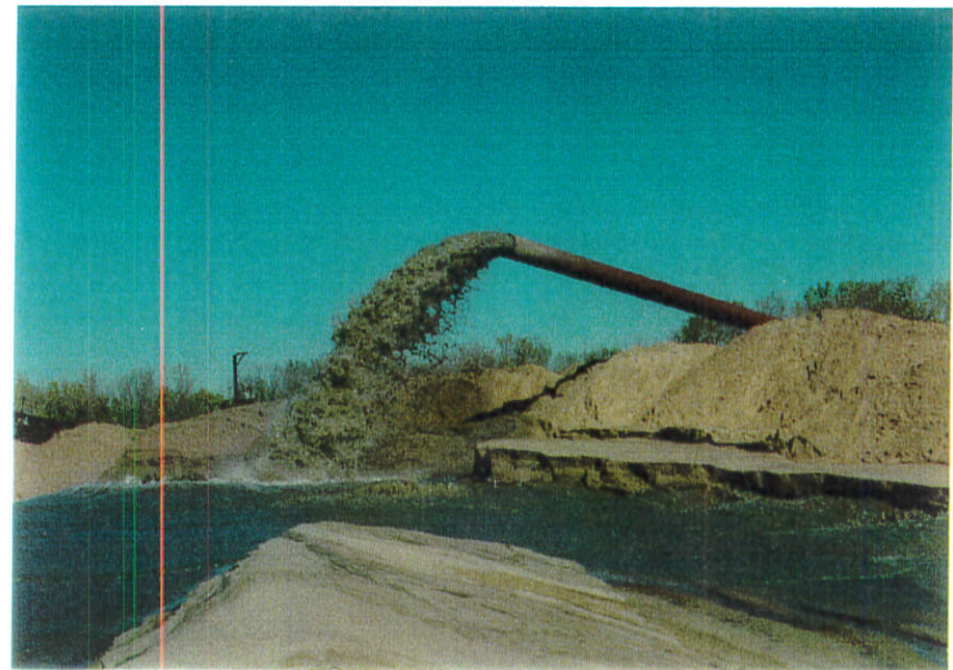
Dredged silt being deposited on land behind holding dikes.
