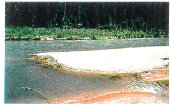
Siltation in upper arm of reservoir.
