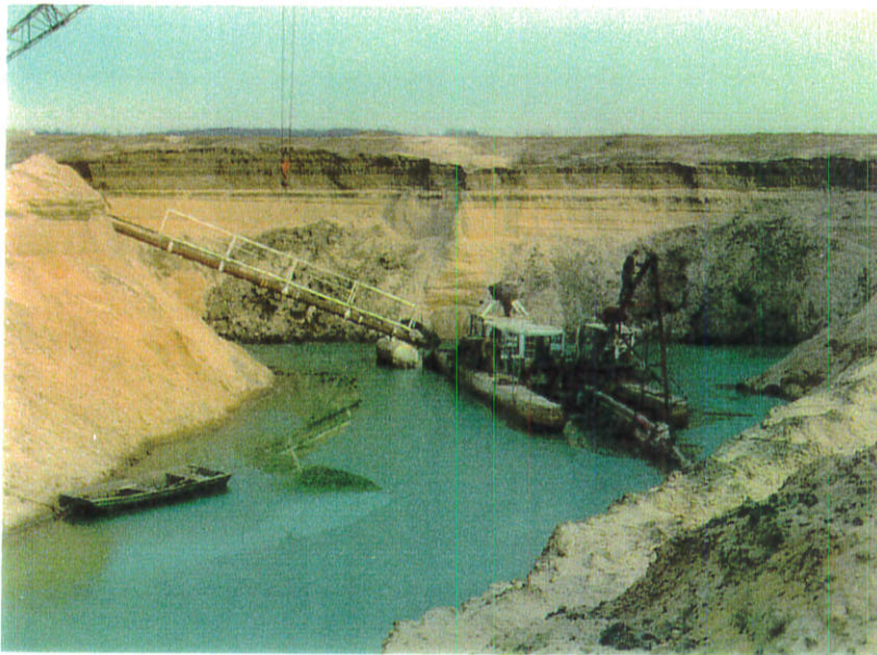
Small basin with siltation and dredging from floating unit.
