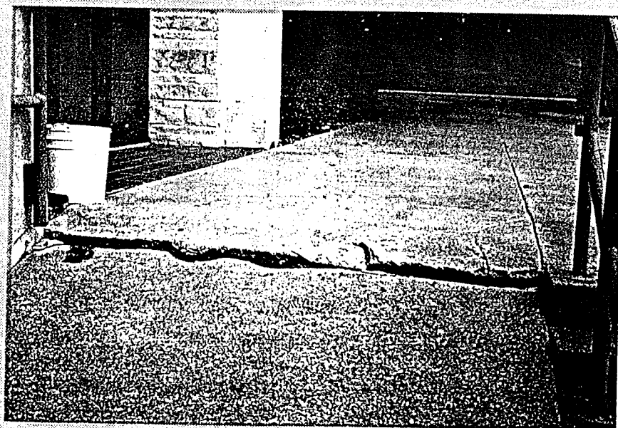
below A settled concrete slab creates a hazard at the front entrance of a KSU building.
