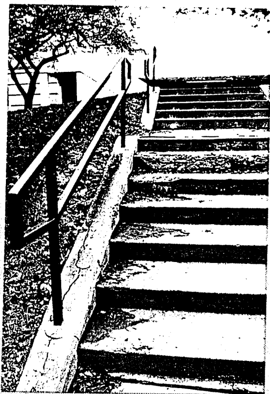
below A settled concrete slab creates a hazard at the front entrance of a KSU building.
