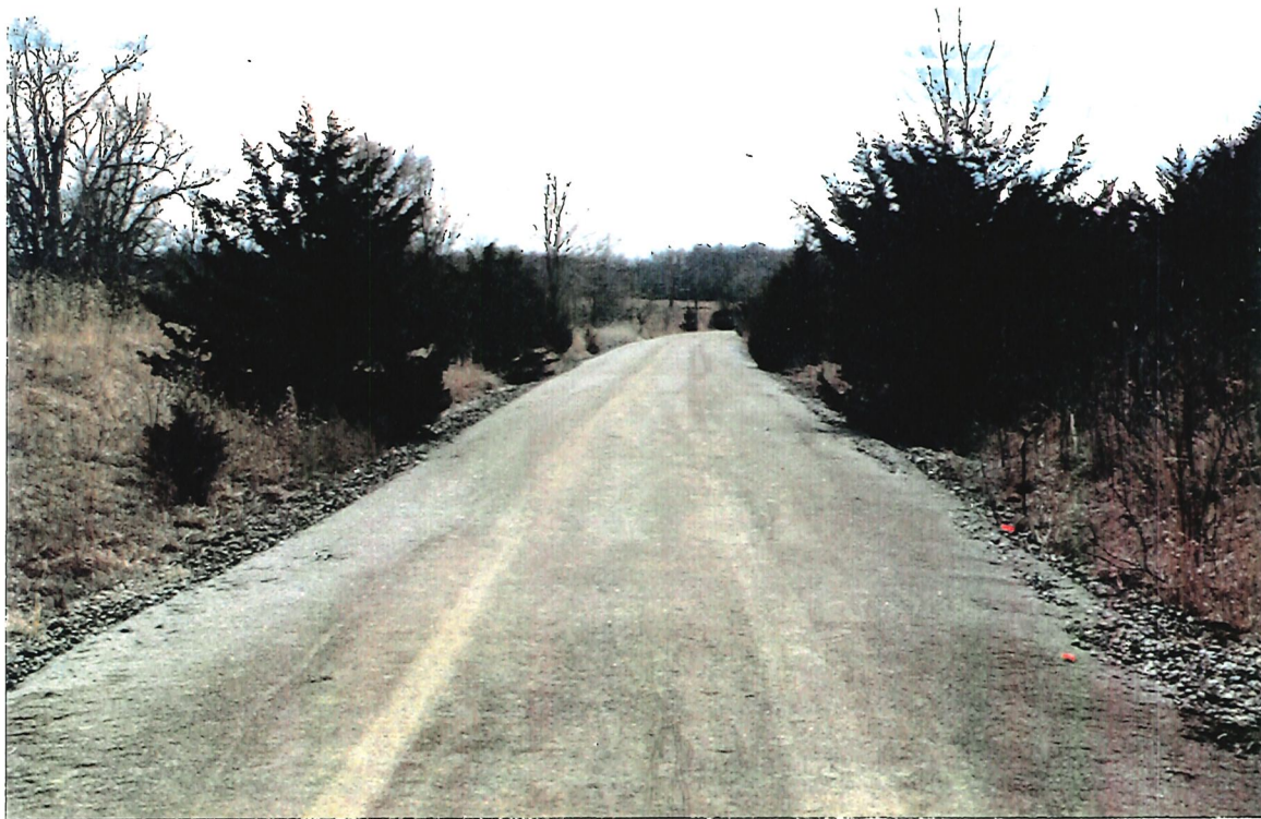
Prairie Spirit Rail Trail: Typical Trail Surfacing
