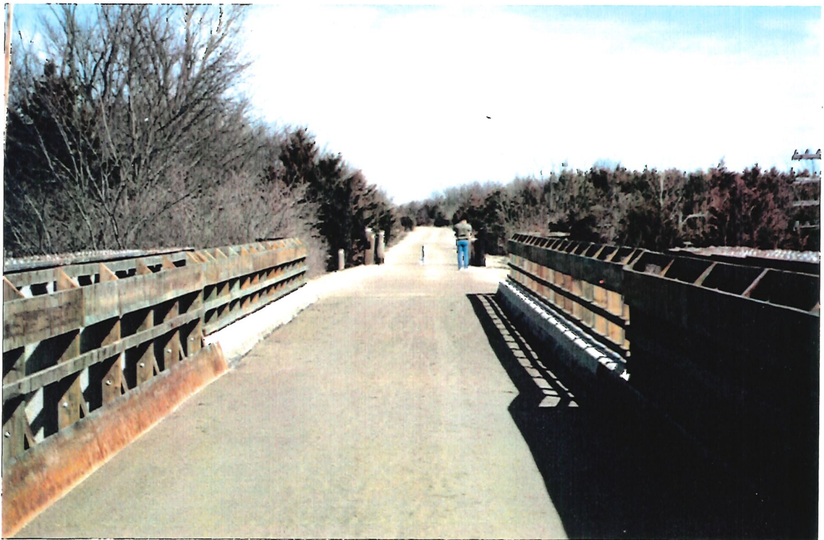
Prairie Spirit Rail Trail: Typical Bridge
