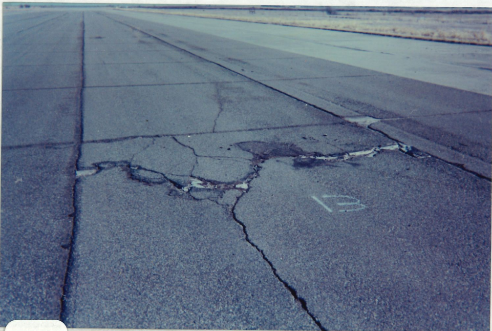
BELOW: Spalled Area Repaired with Oil and Sand Mixture
