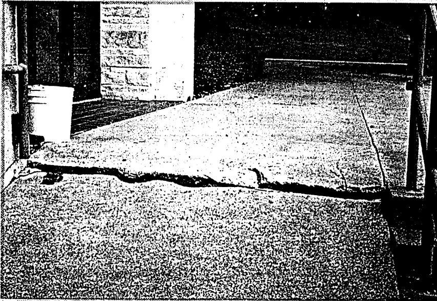
below A settled concrete slab creates a hazard at the front entrance of a KSU building.
