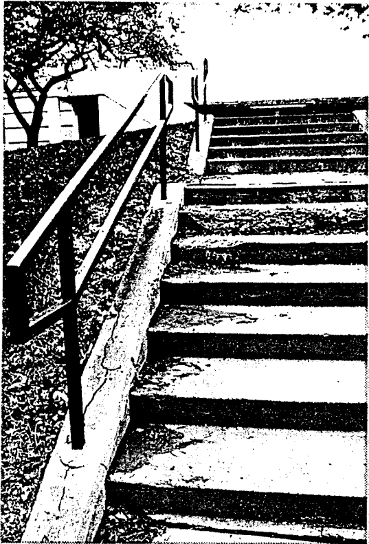
left Steps to Spencer Library at KU are dangerous and unsightly.
