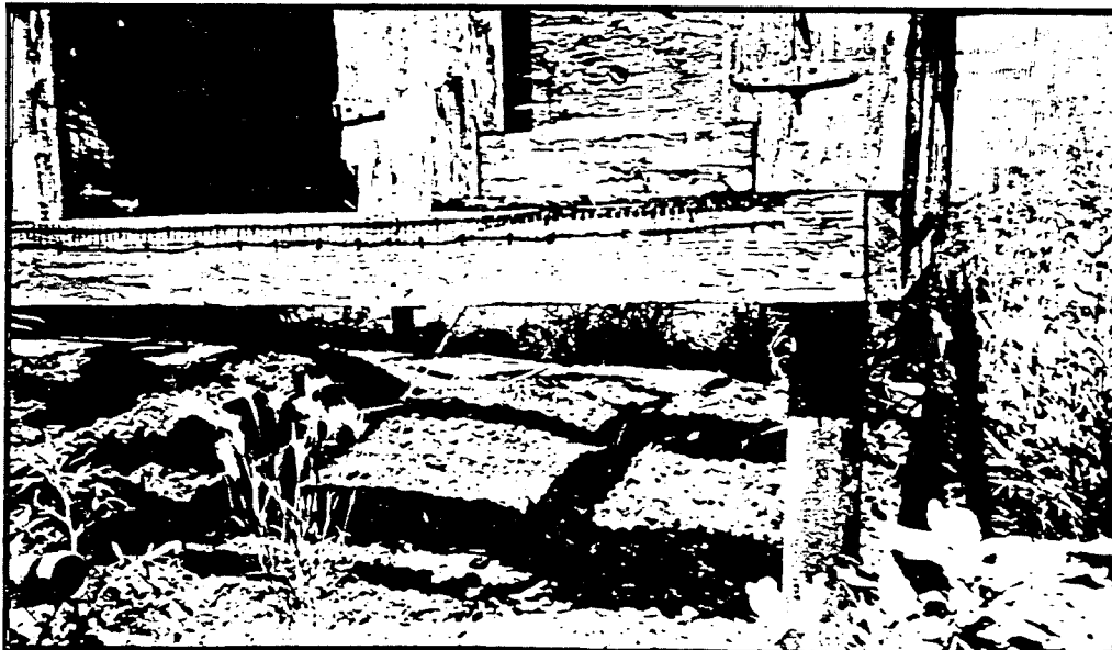
The cages shown at the top of the next page appeared to be of good quality, but no food or water was visible and the area under the cages had not been cleaned out in some time. The middle picture shows what appeared to be a long-dead animal in a wheelbarrow. Finally, the bottom picture shows dogs that appeared to be dirty and in need of grooming. It also shows feces in the cage.
