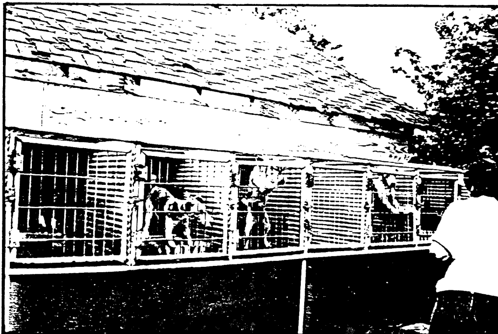
The kennel photographed here also had runs that were built with inside and outside sections. However, unlike the well-constructed building shown above, this facility was in need of paint and general repair.
