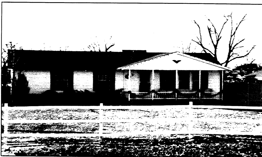
This manufactured house in Osage County has several features which give it a traditional residential appearance, including a double-pitched roof with an eave projection, landscaping compatible with surrounding properties, shutters beside windows, and a carport.
