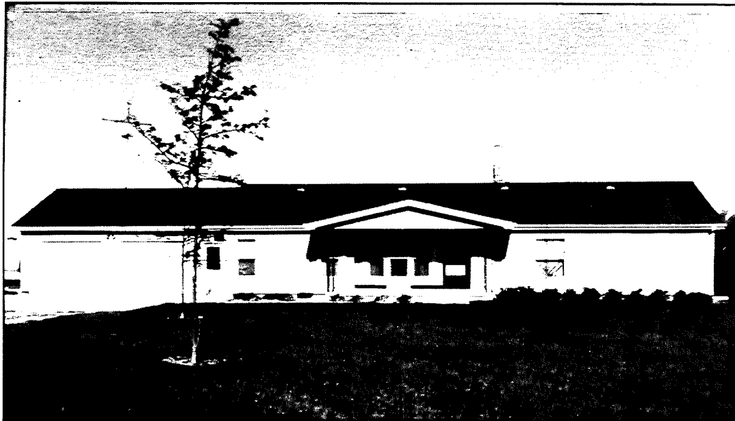
This manufactured house in Ottawa has a doubled-pitched roof with an eave projection, a permanent porch with a pediment style overhang, and an attached two-car garage.
