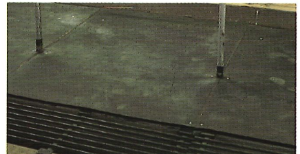
Gutters at the rear of each stall and an automatic scraping system simplify manure handling.
