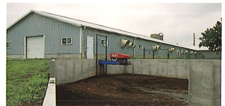
A collection area holds manure until it is spread on nearby fields.
