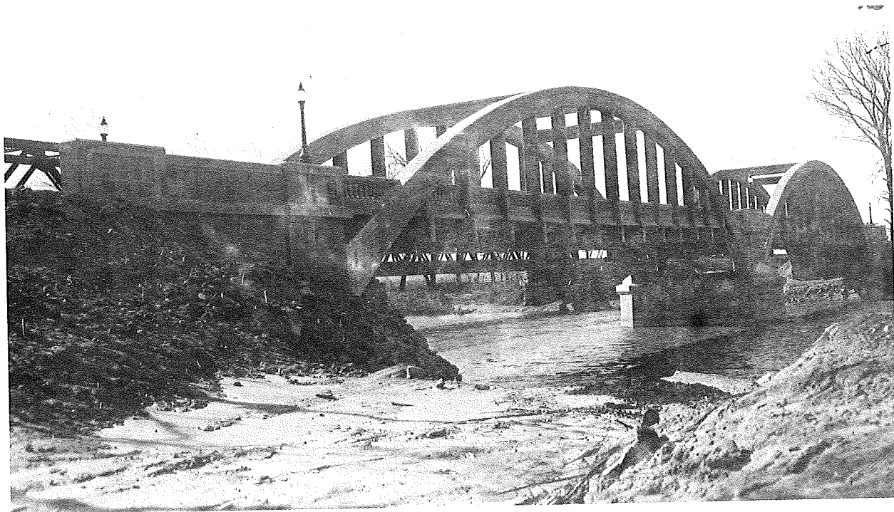
When finished in 1919, the Republican River Bridge near Ft. Riley completed the first federal highway aid project in Kansas.
