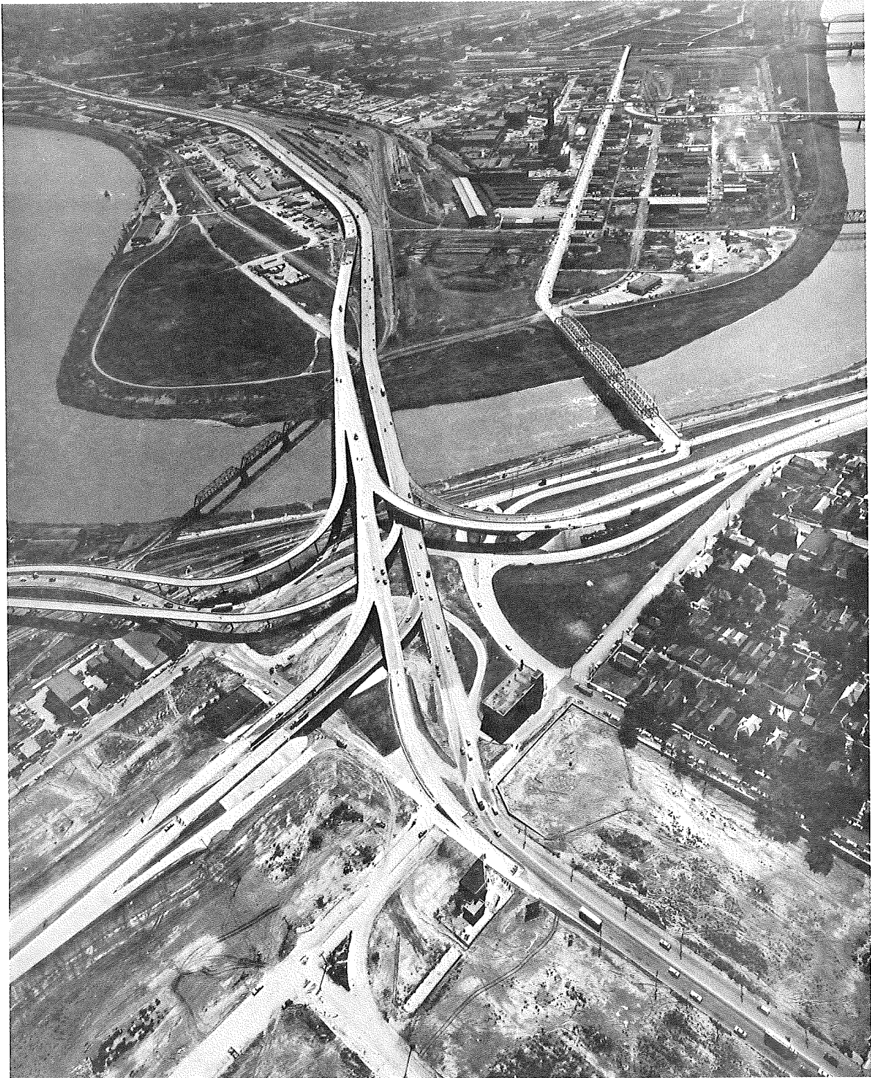
The Lewis and Clark Viaduct linking the two Kansas Citys displays the complexity of design required in the new age of urban highways.
