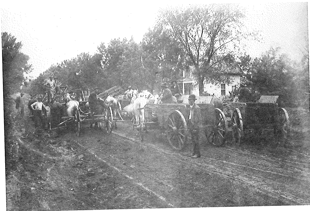
A horse-drawn road grader flattens a rutted Kansas road in 1919.
