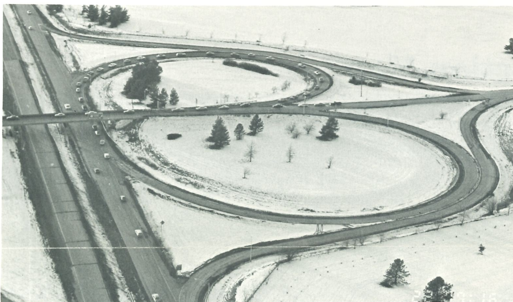
Aerial of I-70 and Wanamaker Exit
