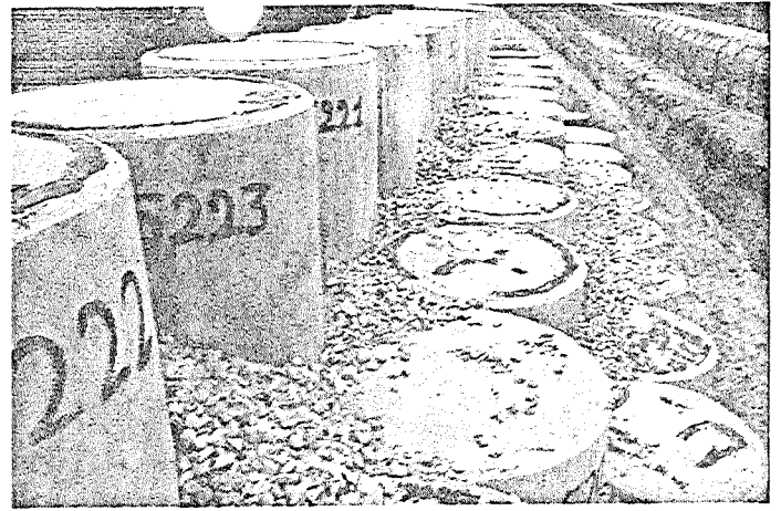
Along the area periphery, the blocks are stacked in a stepped arrangement to give the final tumulus the shape of a gently sloping knoll.
