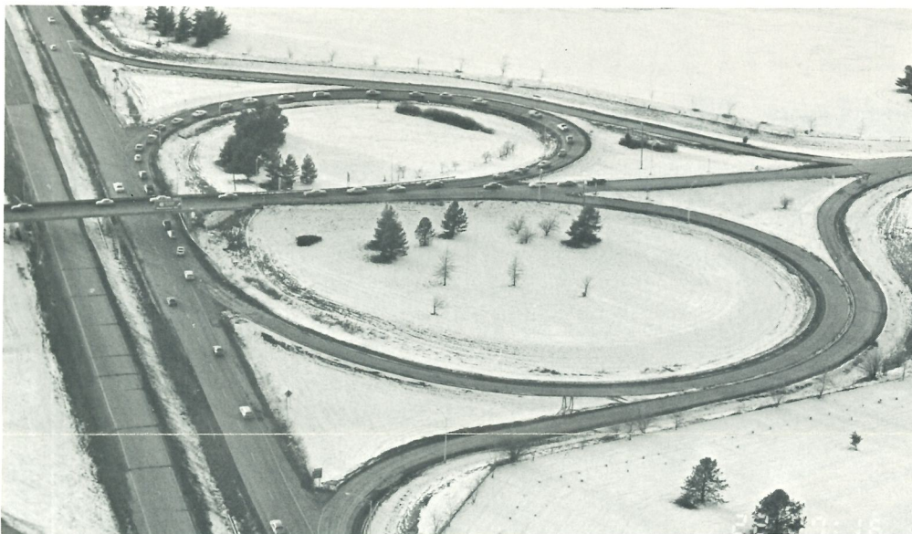
Aerial of I-70 and Wanamaker Exit
