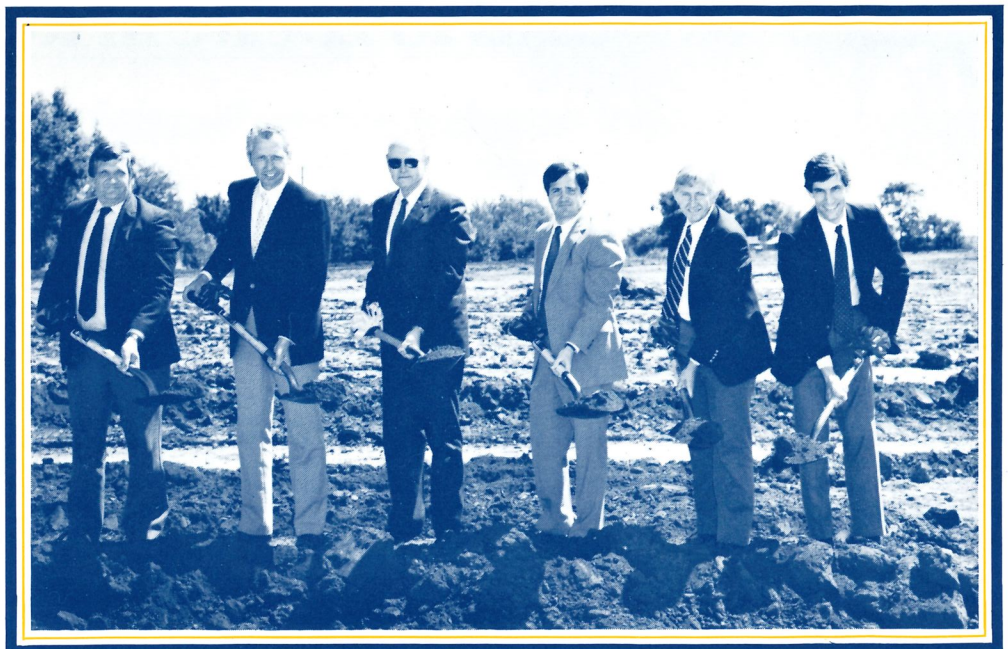
Attending the Northwest Pipe and Casing groundbreaking were, from left to right, Charles J. Schwartz, secretary of the Kansas Department of Economic Development; Steve Gunderson, Idaho First Bank of Boise; Herman Adcox, president of Northwest Pipe; Rich Dickason, president of Atchison Area Economic Development Corporation; Terry Galbreath, general manager for the Atchison plant and Barry Harmon, vice president and comptroller for Northwest Pipe.
