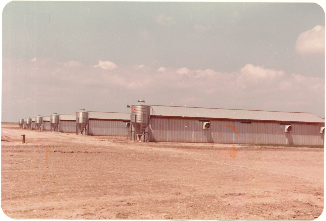
View of Typical Building Construction
