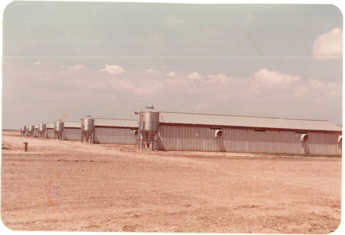
View of Typical Building Construction
