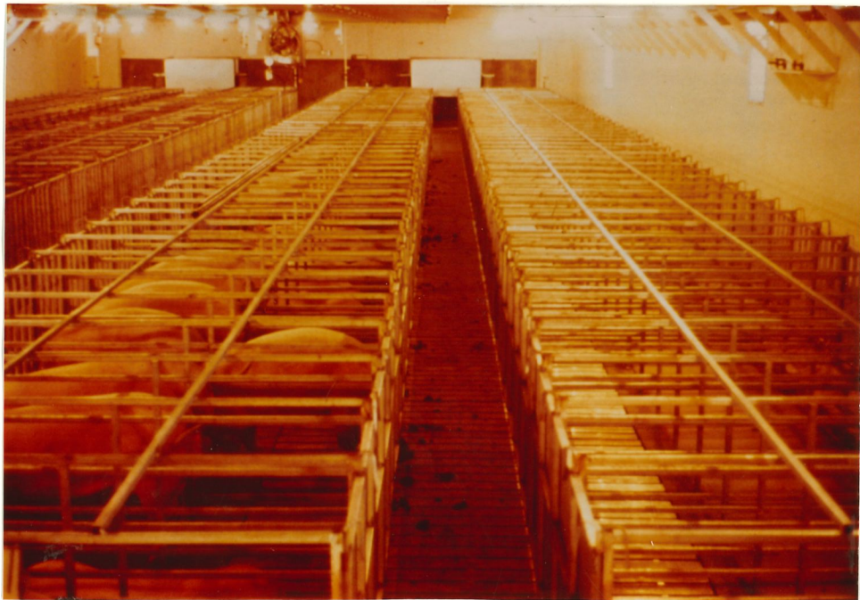
Internal View of Building to show Type of Equipment that could be Constructed by Local Manufacturers
