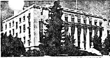
WABAUNSEE COUNTY COURT HOUSE
