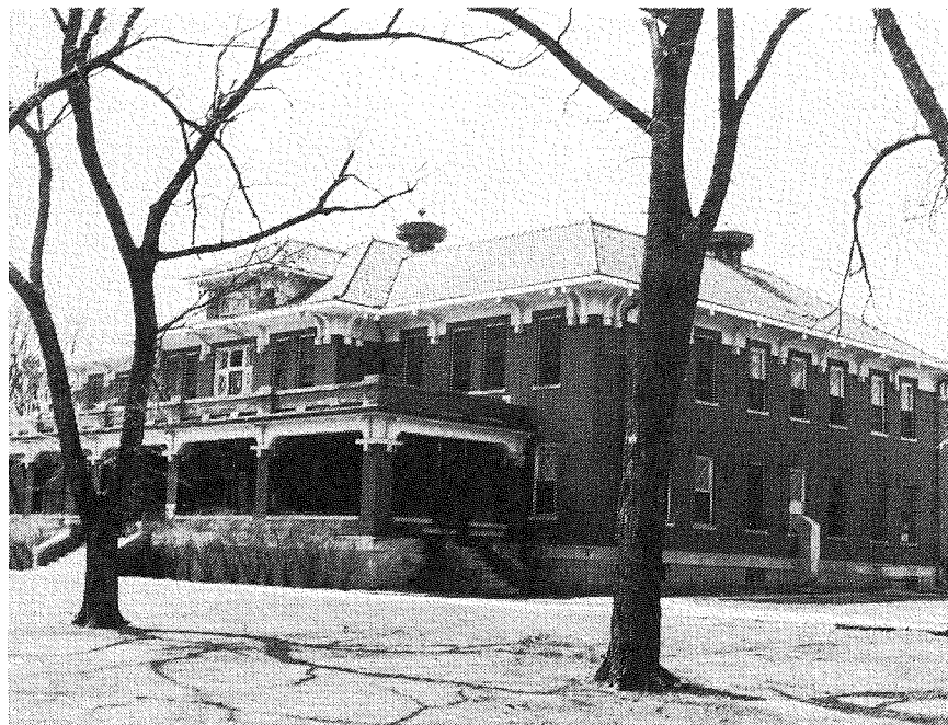
D-Cottage (Perry Cottage) now houses the Staff Library and Nursing Education and other Social and Rehabilitation Services offices. At one time was a unit for female patients.
