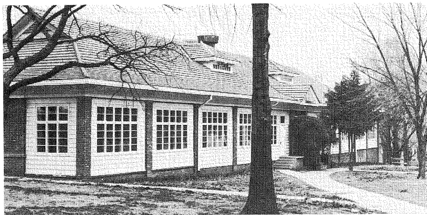
The Tuberculosis Cottage (north of Center Building) has now been razed.
