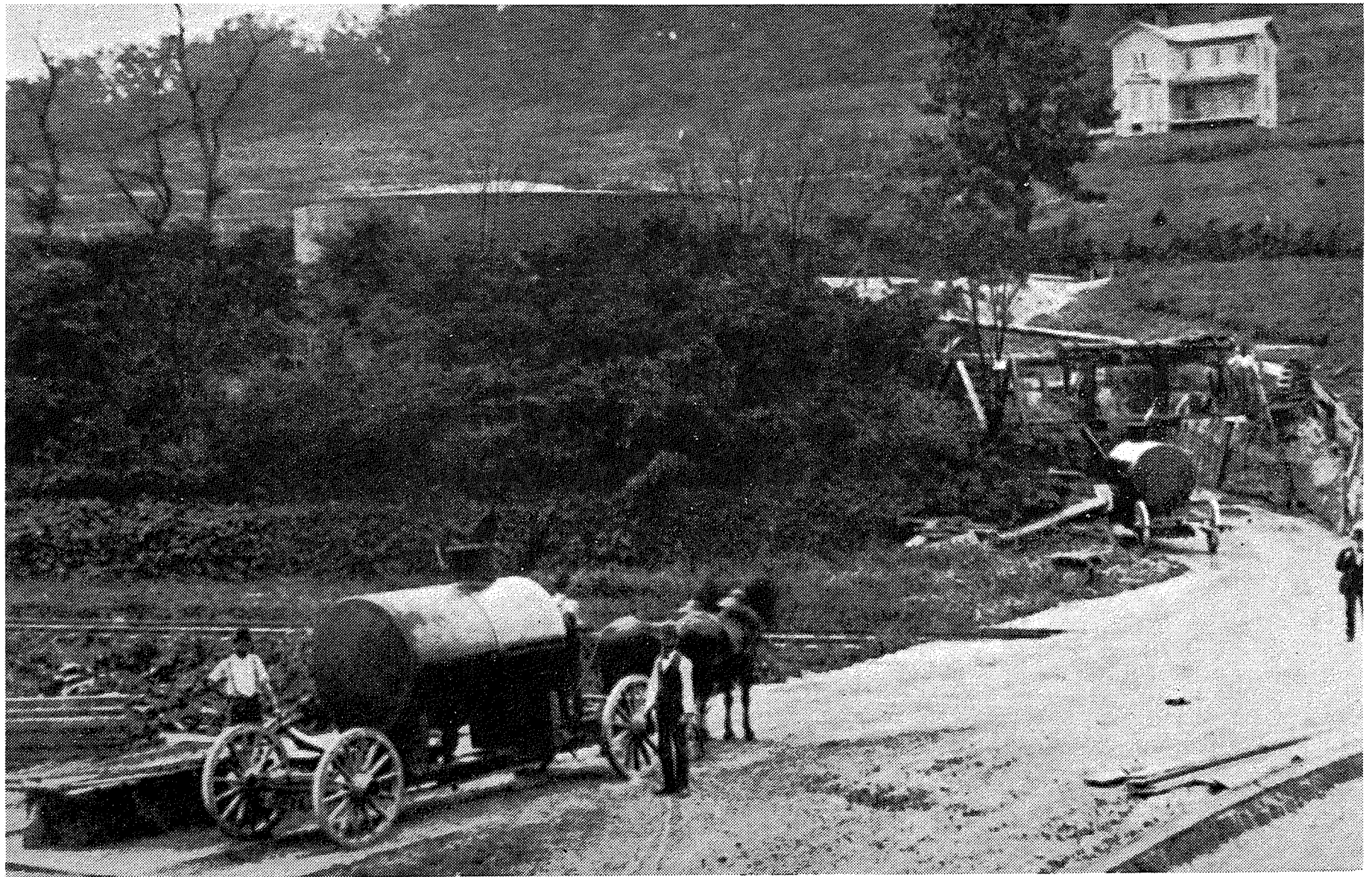
A pipeline challenges a railroad—1875. Denied the right to cross a railroad, Columbia Conduit used tank wagons to move crude oil across the tracks until the court ruled in their favor against the railroad.
