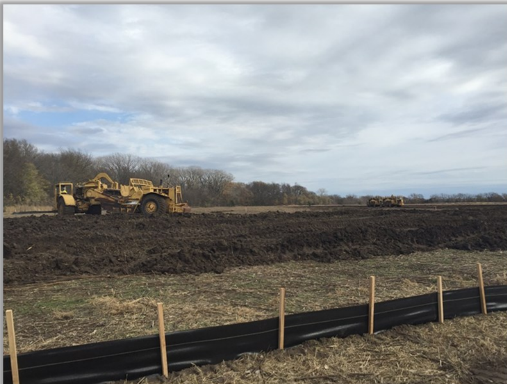
Topsoil removal and placement into stockpiles, CDF B (11/20/2015)
