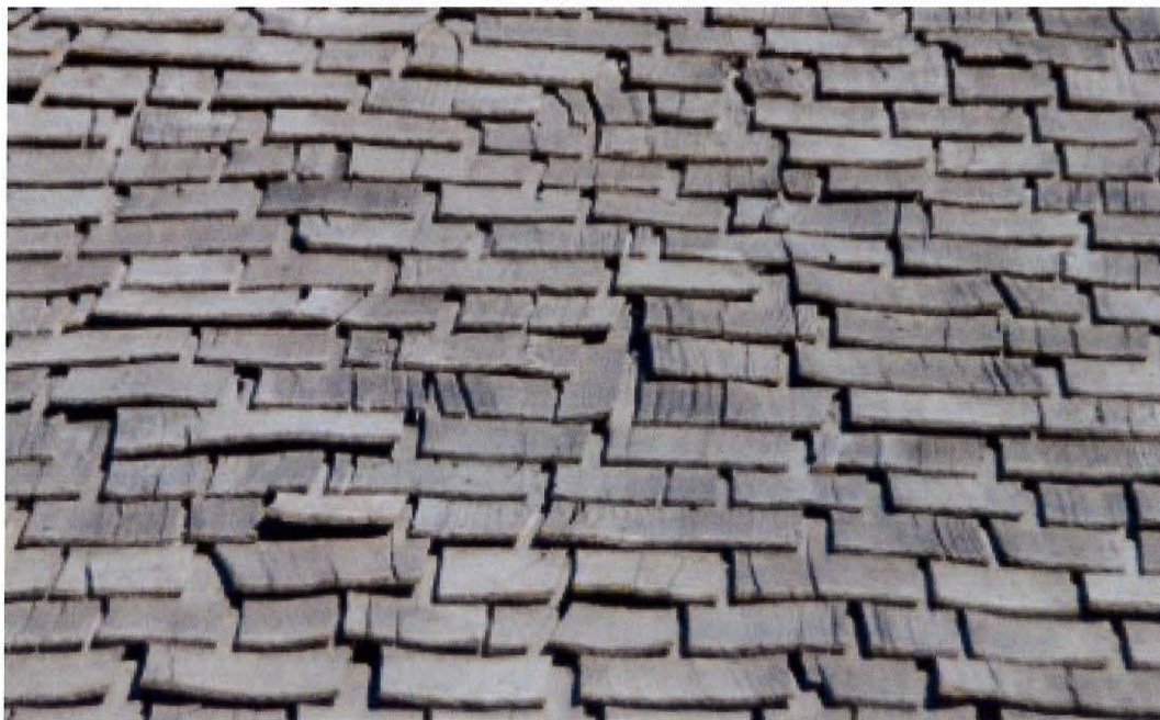
Bunk House deteriorated wood shingles.
