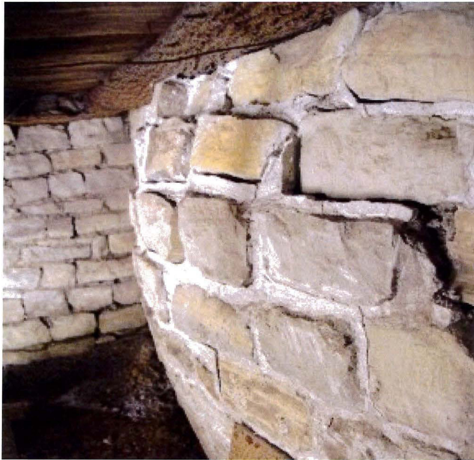
Bulging interior stone foundation wall.
