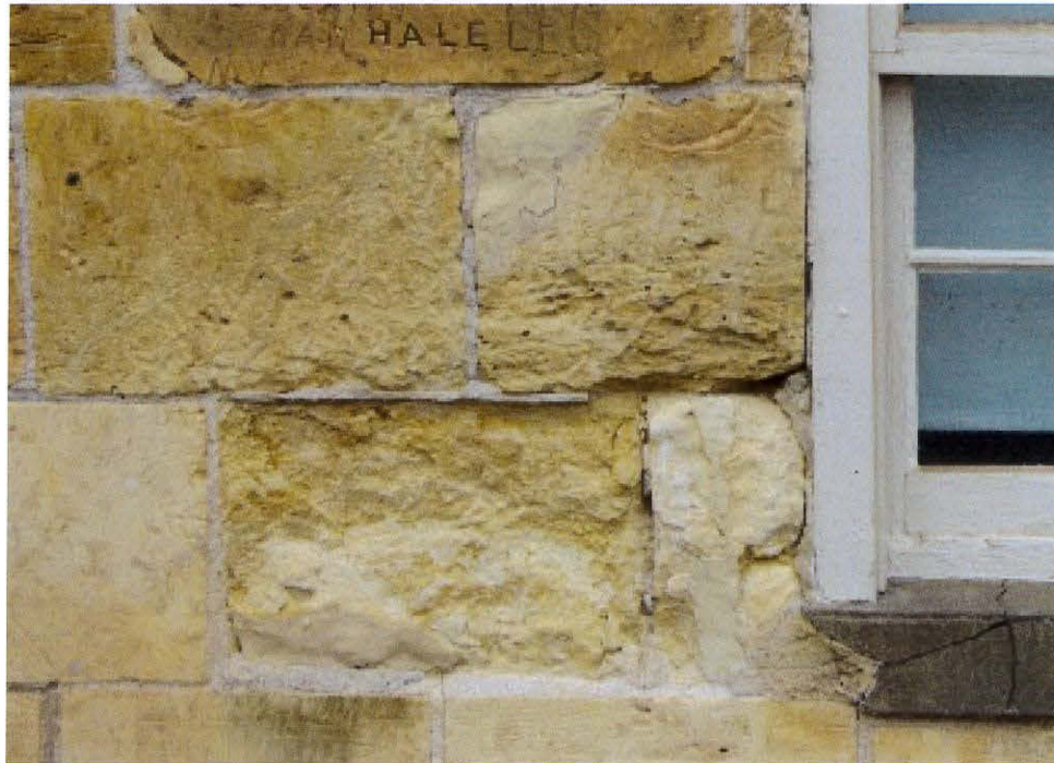
View of deteriorated and spalling stone.
