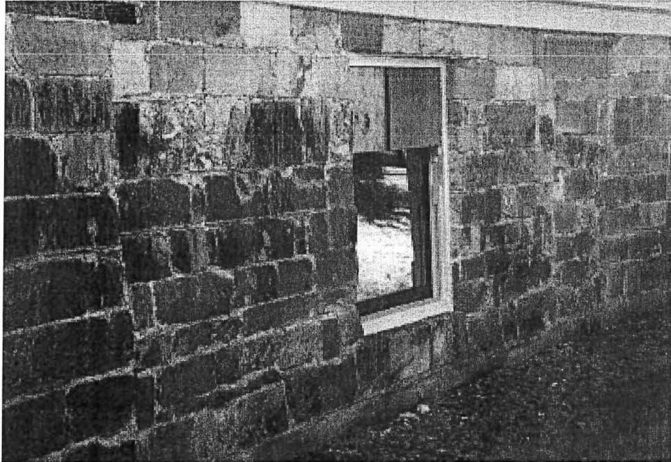
View showing spalling and cracked stones.
