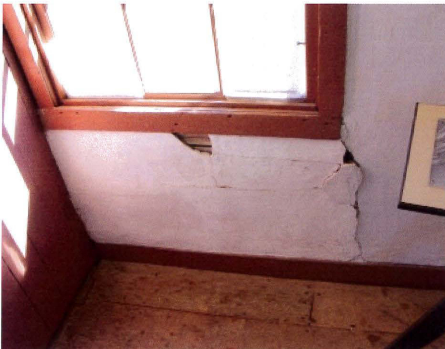
View of interior plaster damage.
