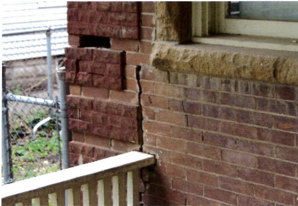
View showing missing brick and displaced corner.
