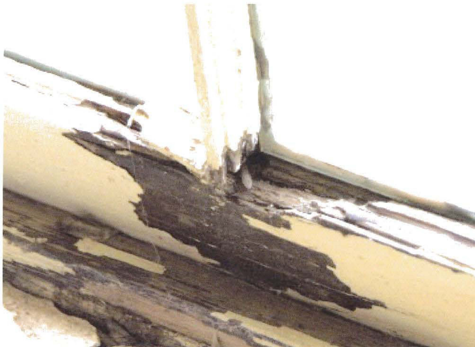
View of deteriorated window frame.
