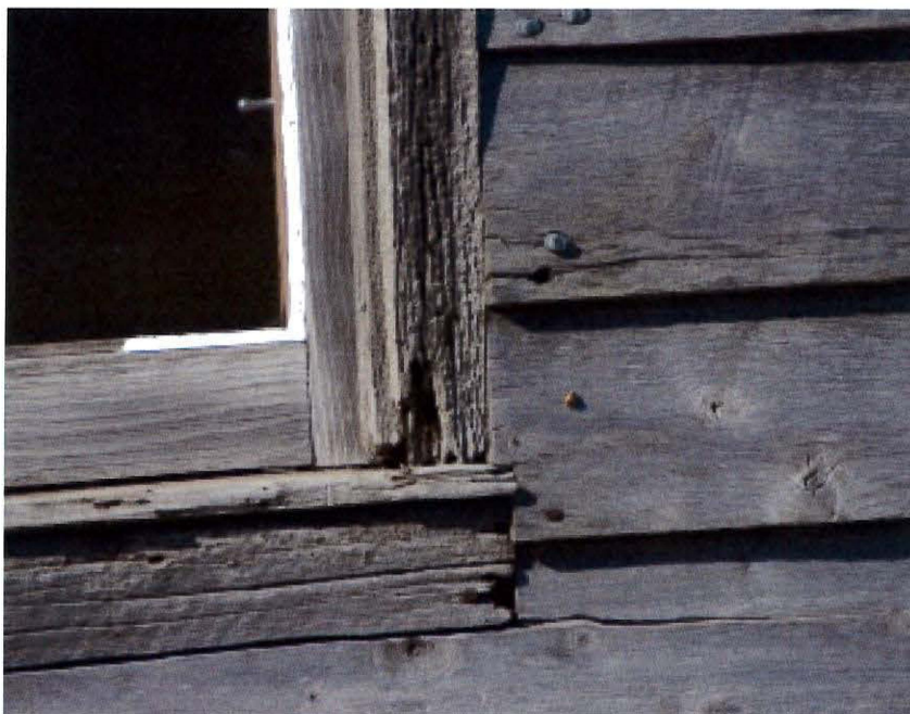
View of deteriorated wood trim.
