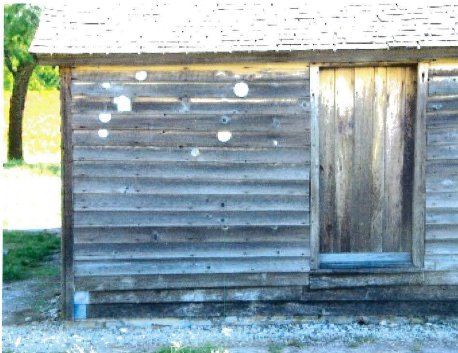
View of partial west elevation damage and temporary repairs.
