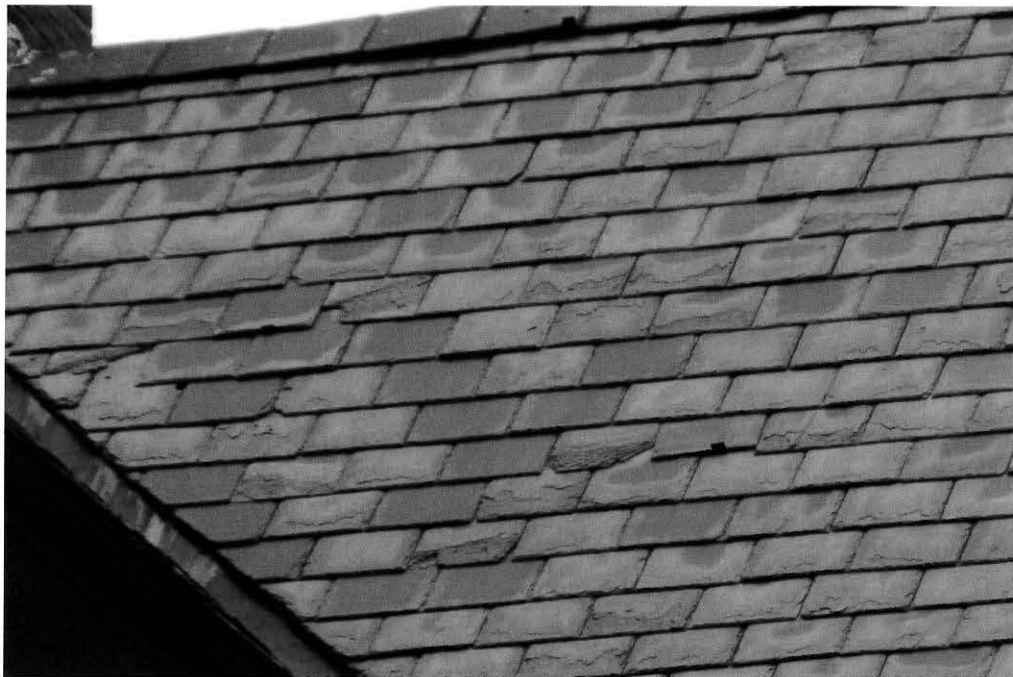
Delaminated and broken slate.
