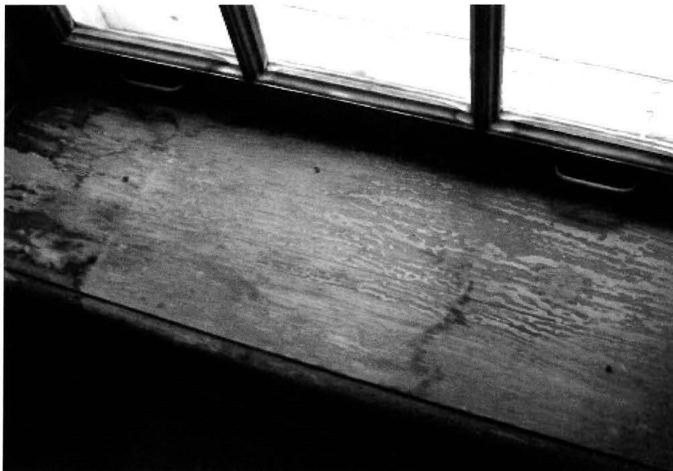
Damaged interior wood finishes.
