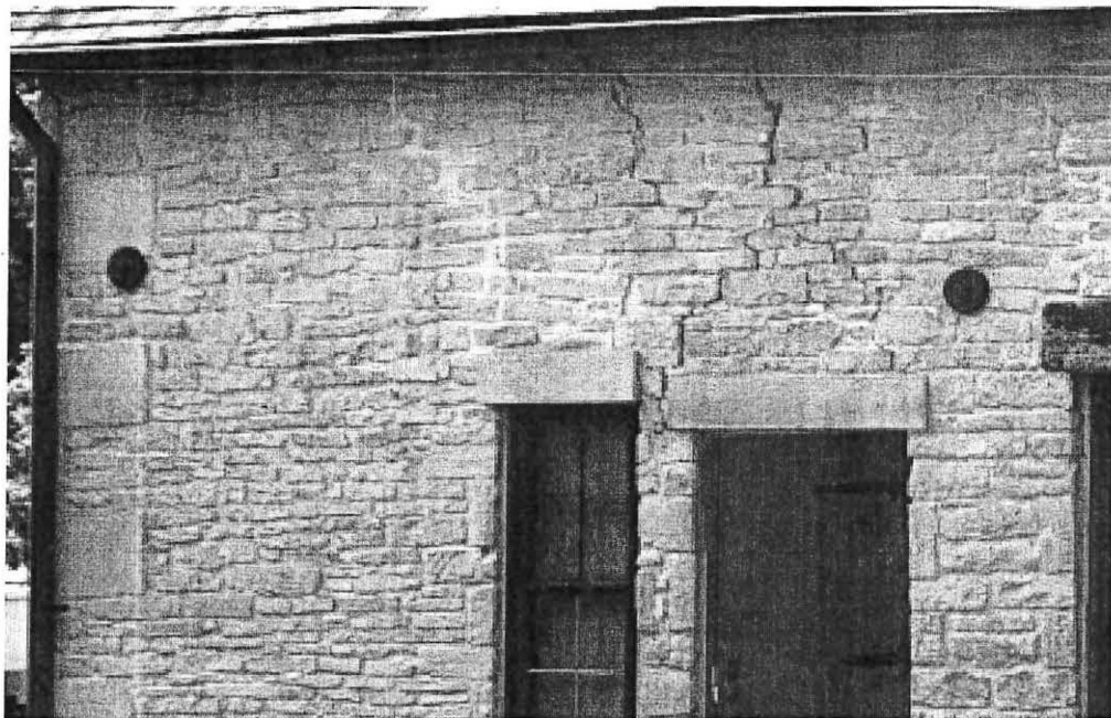
Cracks showing shifting of north wall.
