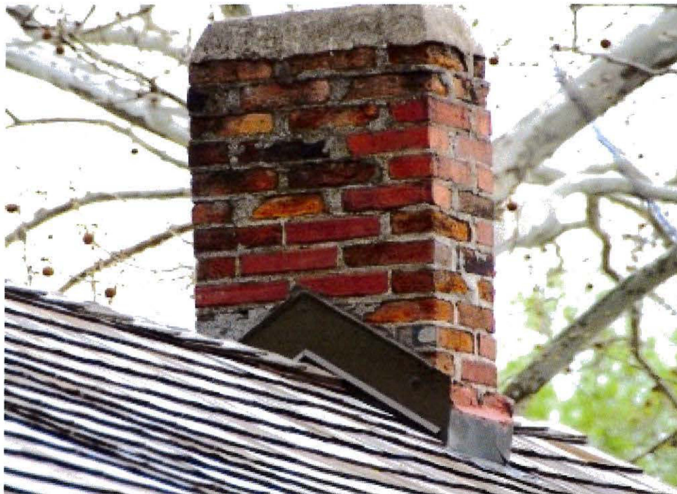
Brick chimney with damaged and spalling brick.
