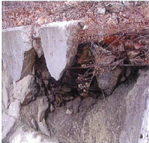
Damage to spillway
