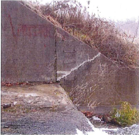
Damage to drop structure under bridge
