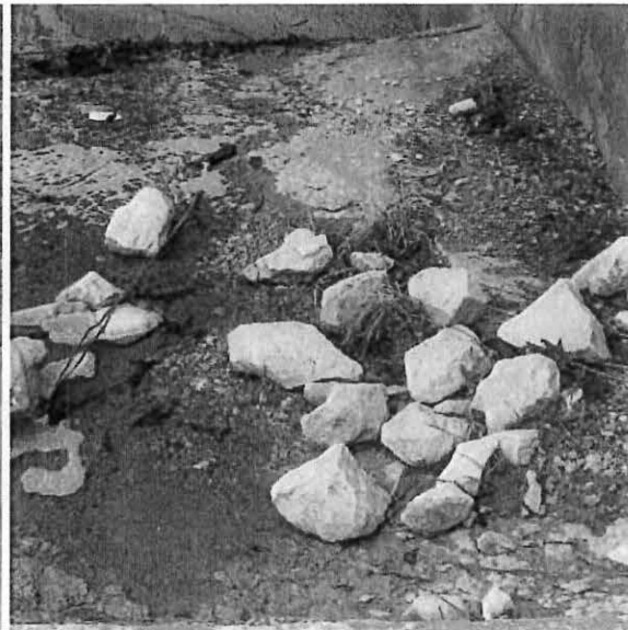
Concrete Damage to weir floor
