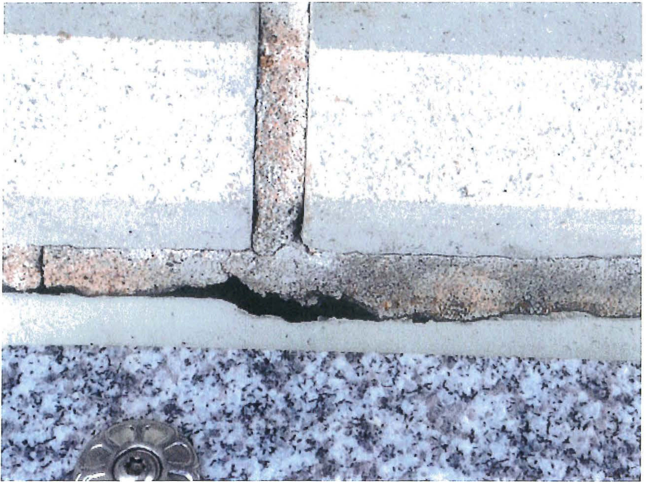
Winfield Cemetery Repair Loose Building Mortar Close Up Detail of an Example of the Repairs Needed
