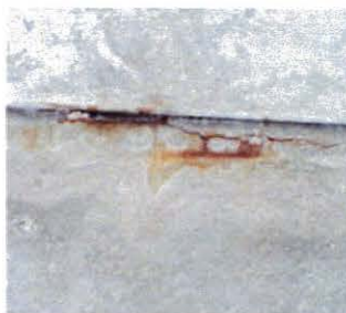
Corroded Double T Flange
