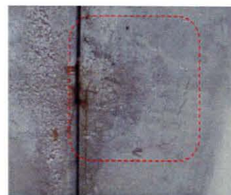
Spalling double T Flange
