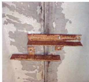
Rusted Shear Connectors
