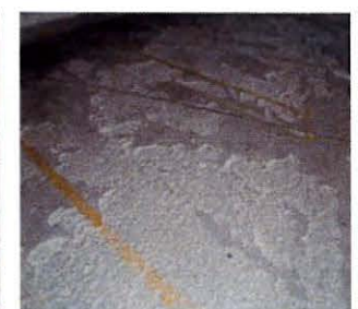
Concrete Scaling
