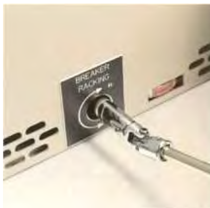
racking access port with front door closed.
