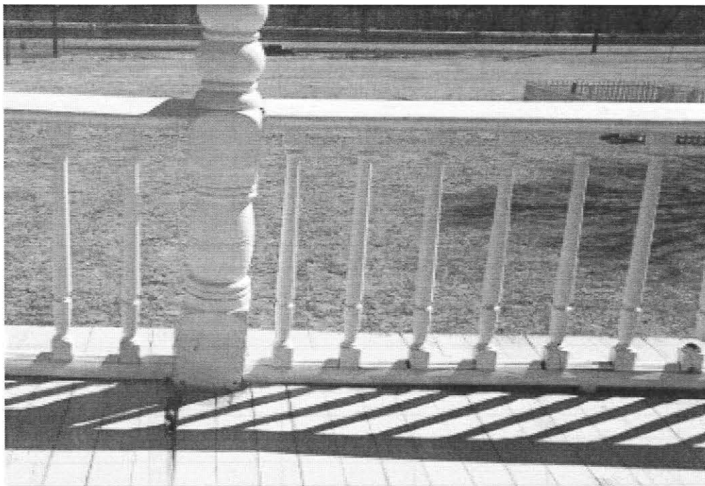
View of wood column sunken down into deteriorated wood decking
