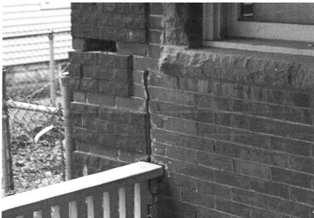
View showing missing brick and displaced corner
