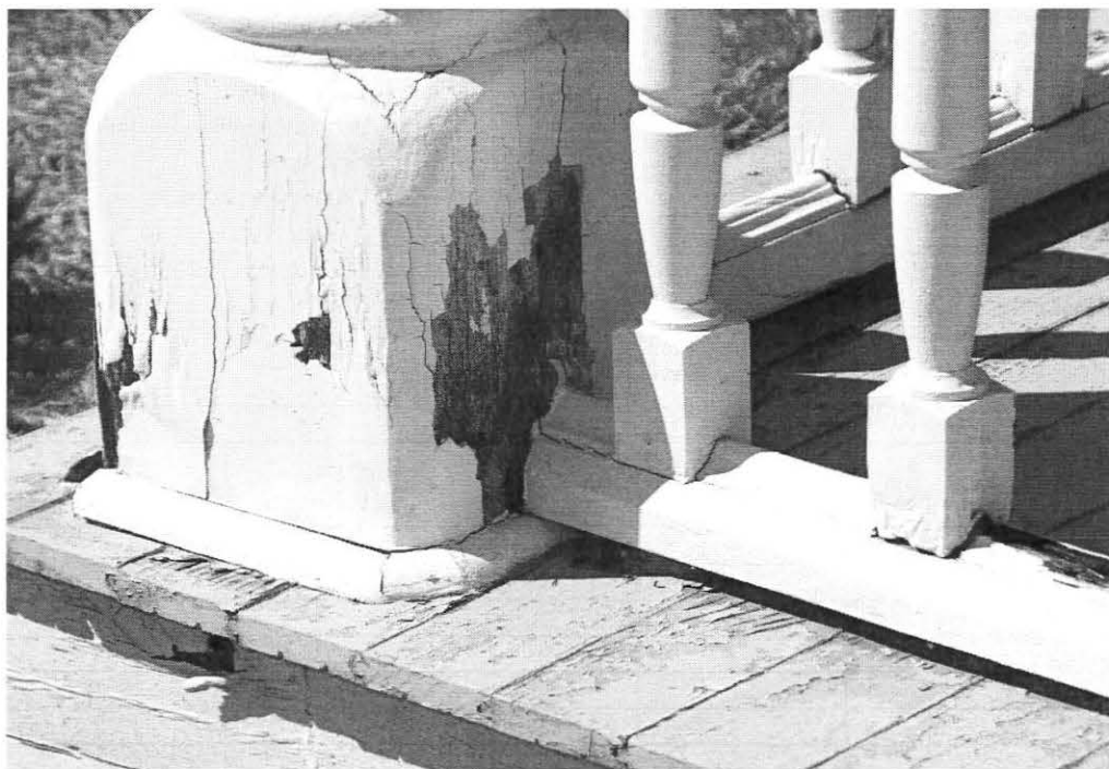
View of deteriorated column base and railing balusters
