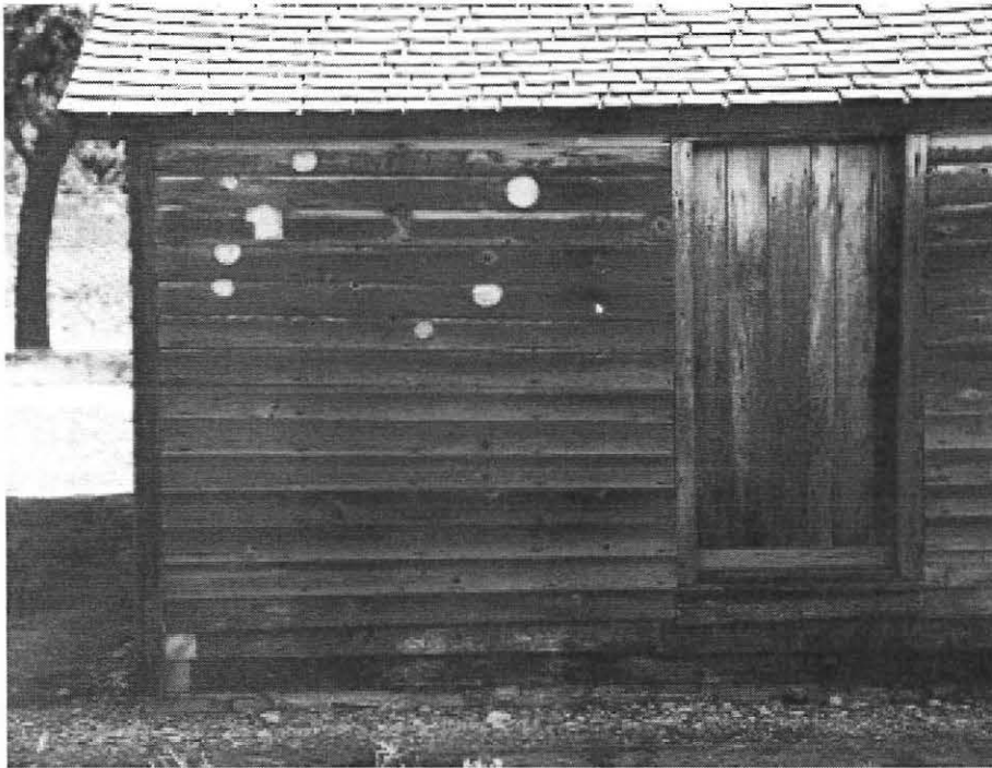
View of partial west elevation damage and tempory repairs
