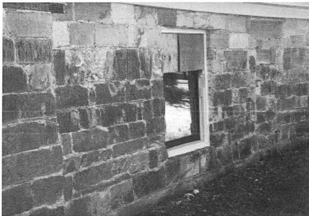
View showing spalling and cracked stones
