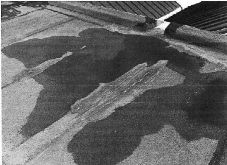
View of section of roof has separated from the substrate below
