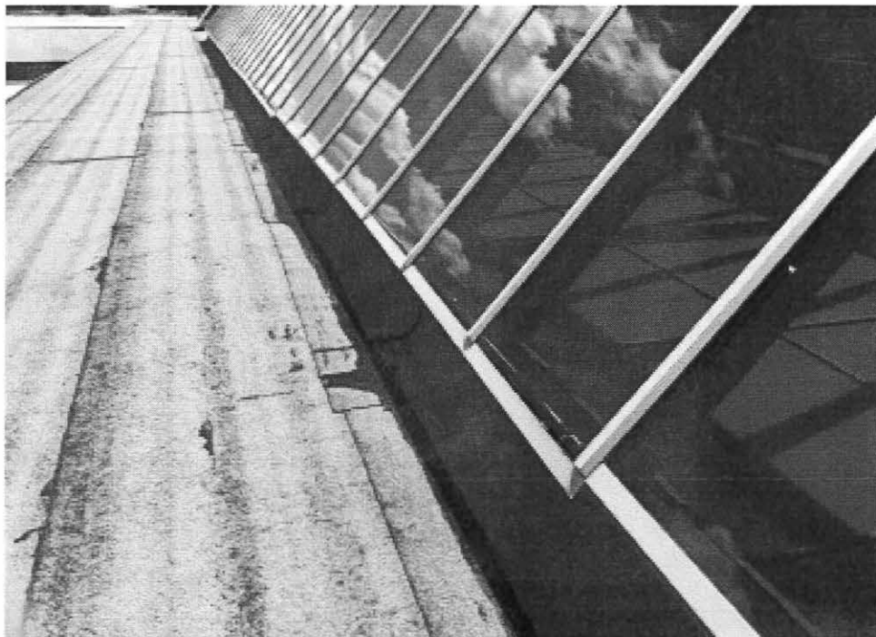
View of flashing on skylights that needs repair
