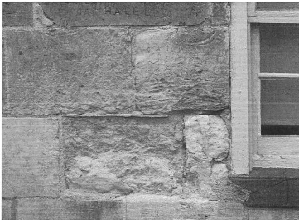
View of deteriorated and spalling stone
