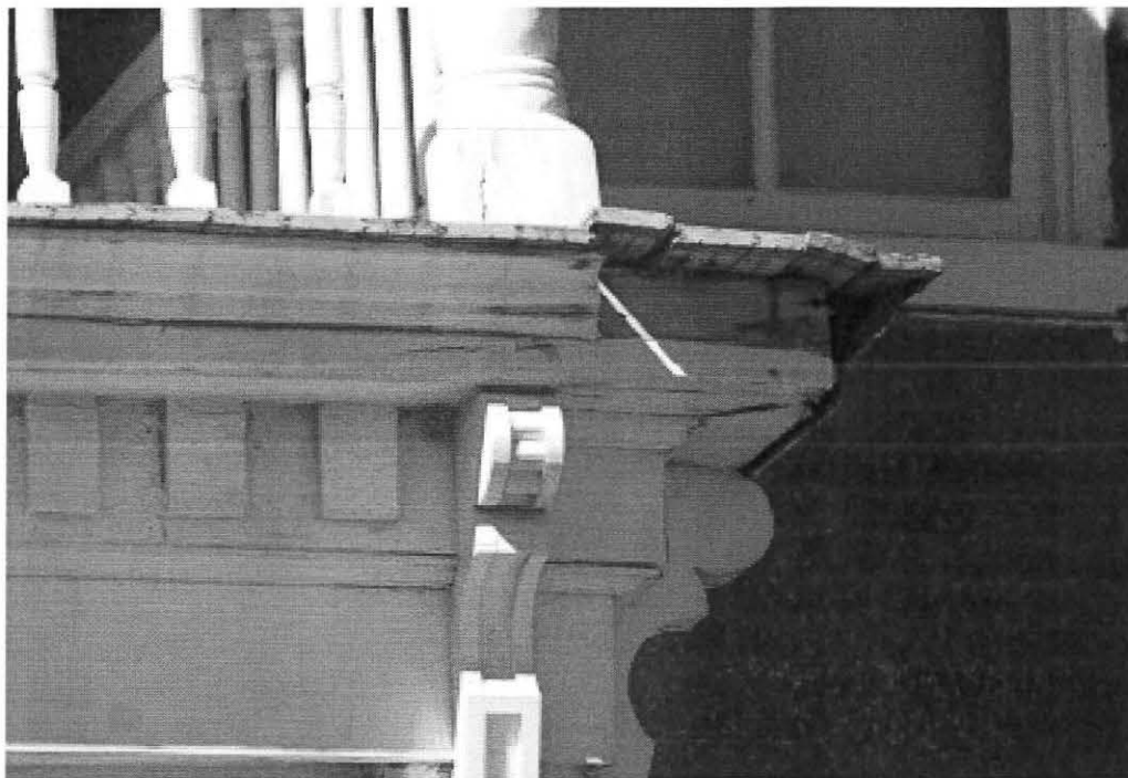
View of deteriorated crown molding and porch deck
