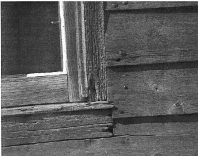
View of deteriorated wood trim
