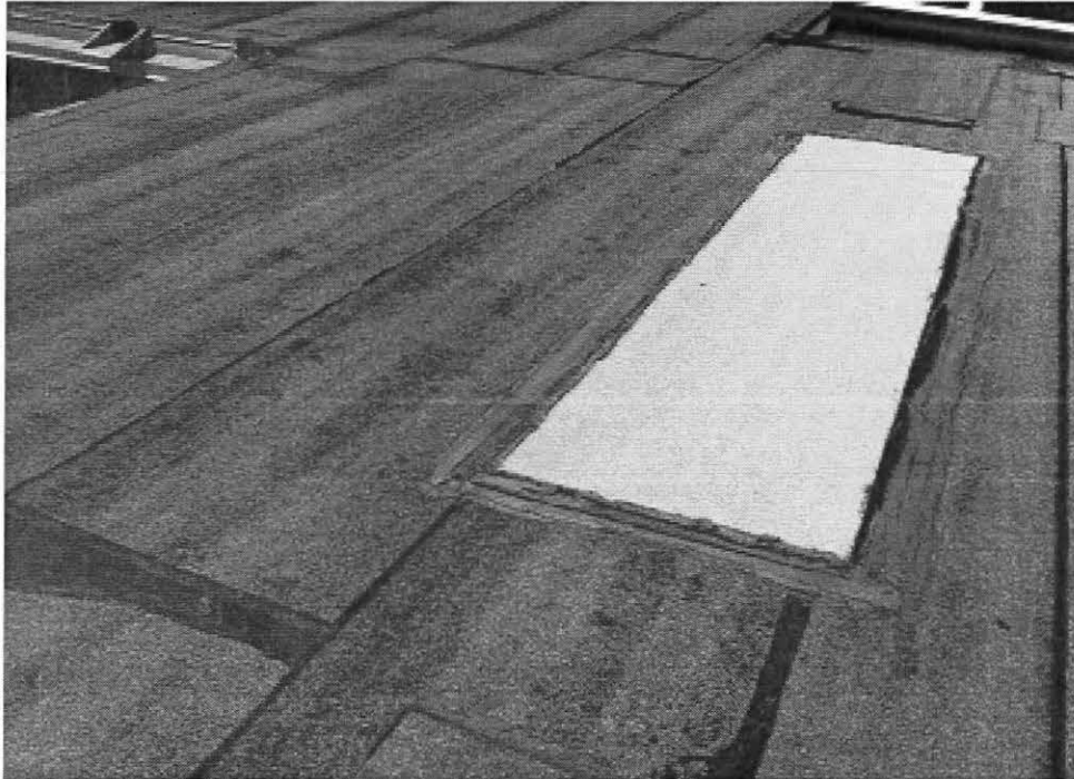
View showing loss of protective granular surface and patching
