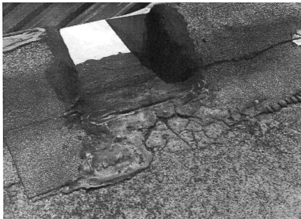
View of previous patching that is failing
