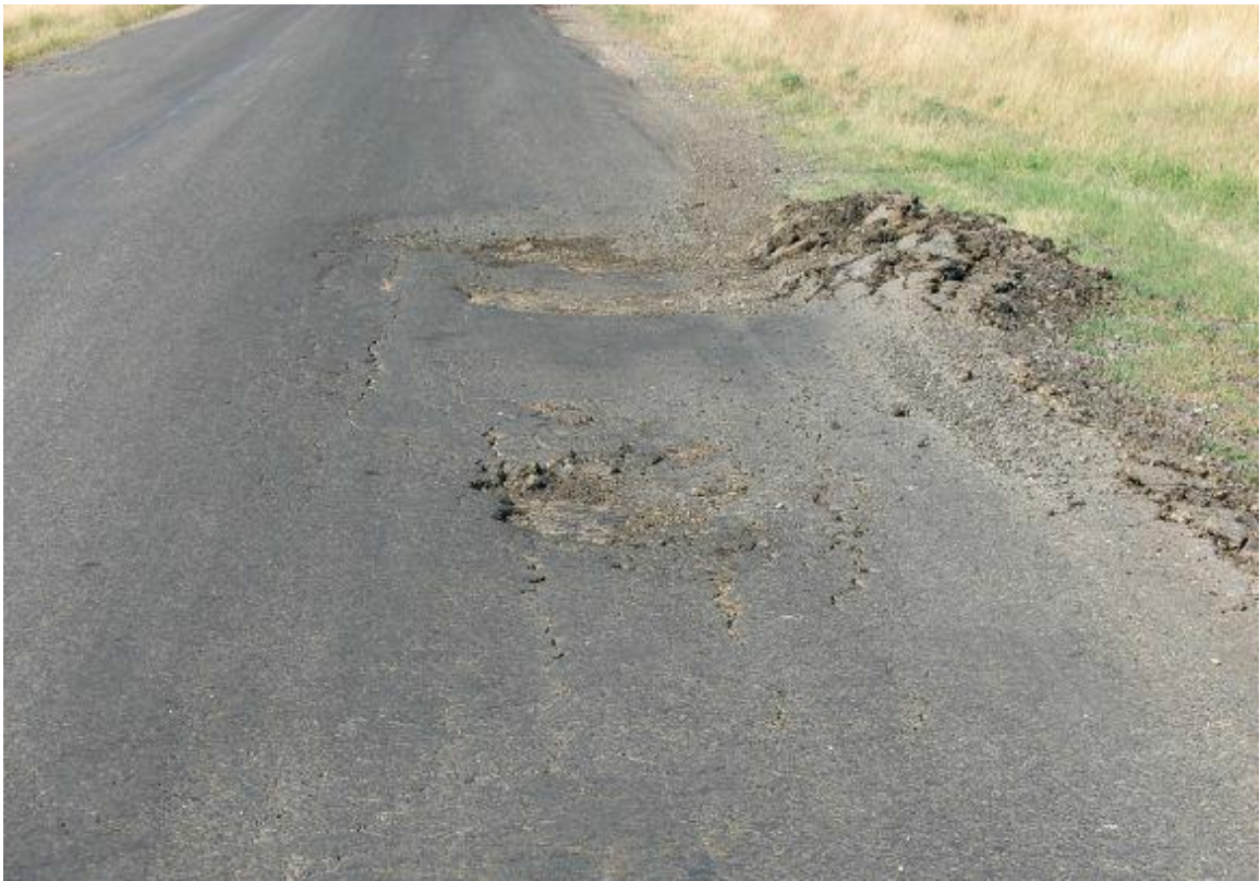
Figure 4 Potholes and ruts caused by heavy loads may be a safety issue for autos.
