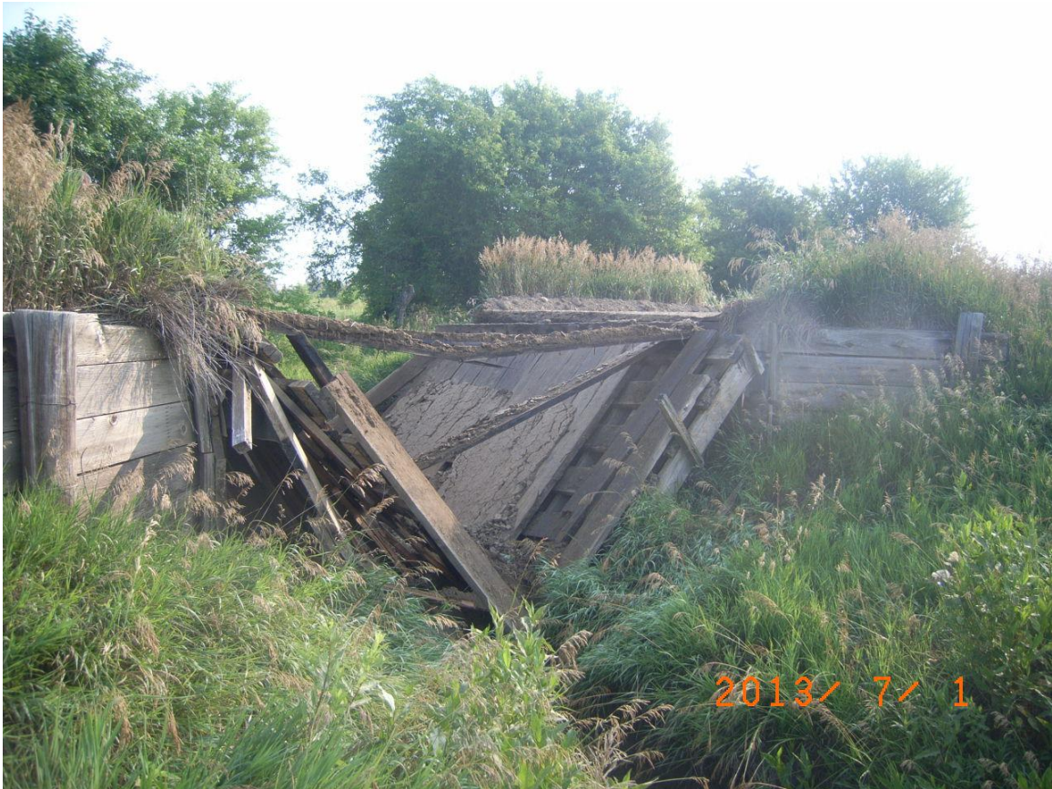
Figure 6 Another timber bridge collapse due to overweight
