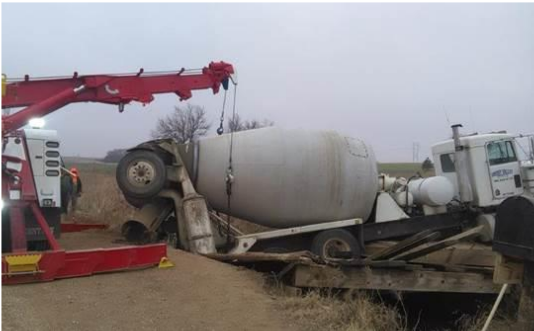
Figure 5 Timber structure collapse
